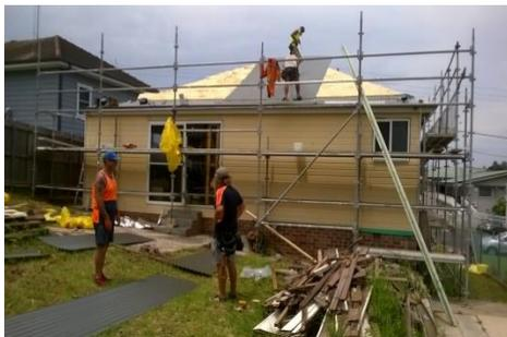
Currently the exterior has been totally repainted by volunteers, all interior framing completed, all walls and ceilings insulated, all first fix electrics and plumbing as well as NBN wiring completed.
